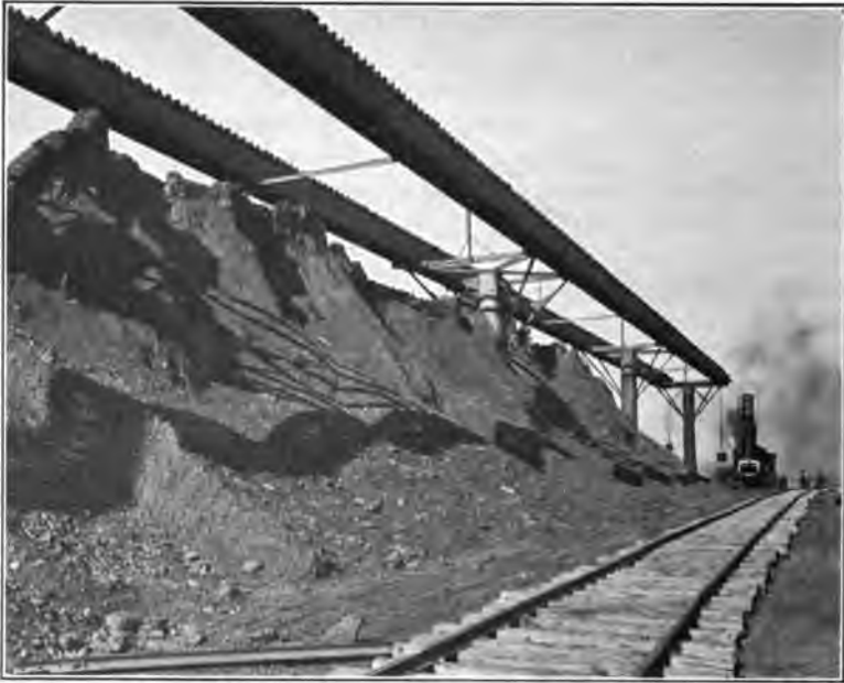
STOCKPILE AFTER REMOVAL OF ONE CUT BY SHOVEL
